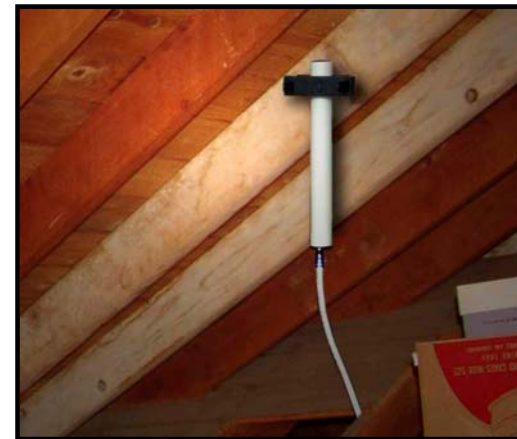
Figure 5 - Mounting Signal Antenna to a Main Beam
